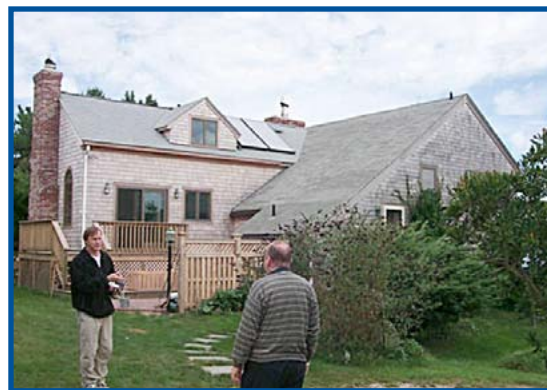
PV provides year round solar-assisted power to a domestic water-heating system for this residential addition in Rhode Island. Photo courtesy of NREL.
